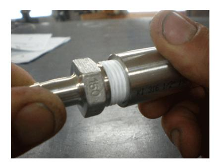
Insert into female fitting, make sure thread is located properly and tighten until sealed. Be careful not to wind the fitting back at all, as the tape is a 'one shot deal' and if you undo it it may not seal properly and you will have to re-tape it.
